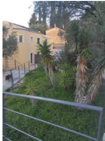
Railings finishing off
