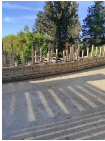
Top wall shuttering
