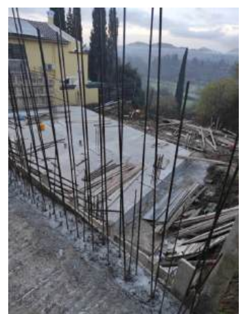
Steel for upper retainer
