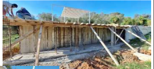
Shuttering extended pool area
