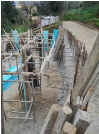
Steel lining wall to be
