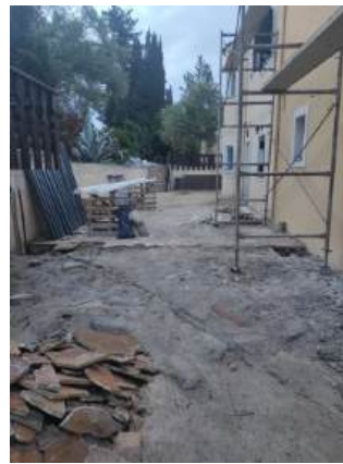
Paving, paving, and paving
