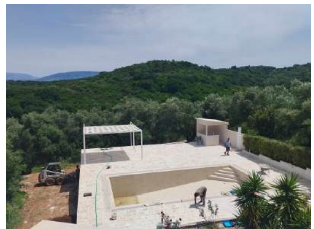
Working on the pool
