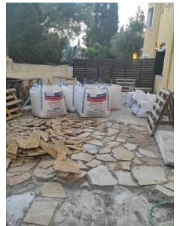
I thought that paving would never finish
