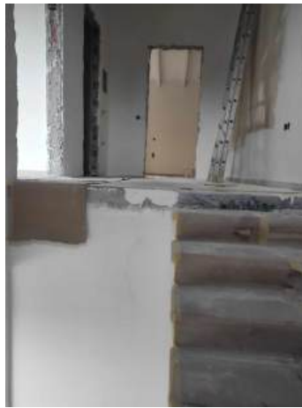
New upper storey almost there
