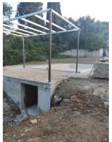
Working area being tidied
