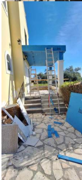
Widening of entrance
