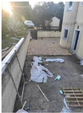
Crazy paving former concrete area
