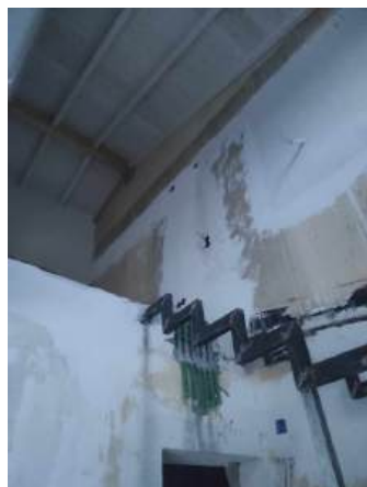
New stairway going in to new storey
