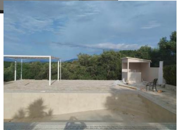
Pool area with kiosk taking shape
