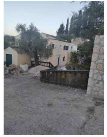
Part of new wall at front
