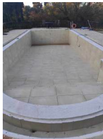
Old pool newly tiled
