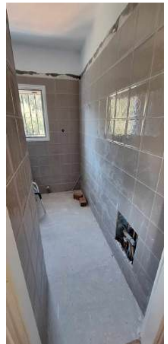
New tiling throughout villa
