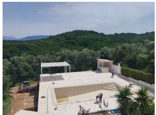
Working on the pool
