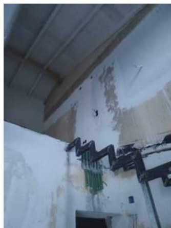
New stairway going in to new storey
