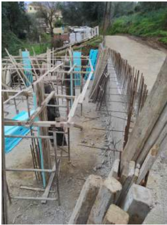
Steel lining wall to be
