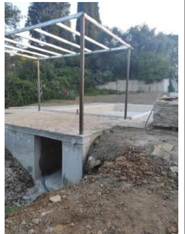
Working area being tidied
