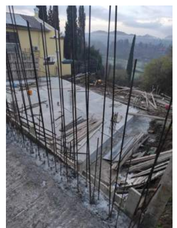
Steel for upper retainer
