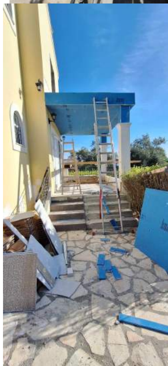
Widening of entrance
