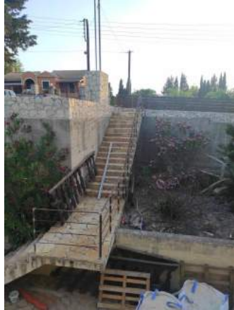
New steps to the road
