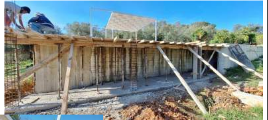
Shuttering extended pool area
