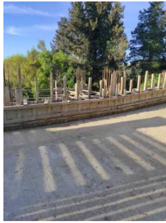
Top wall shuttering
