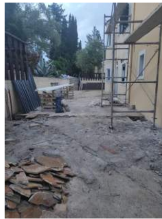
Paving, paving, and paving
