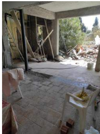
This used to be a nice lounge
