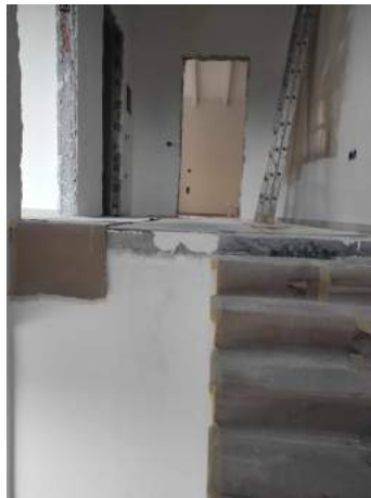
New upper storey almost there
