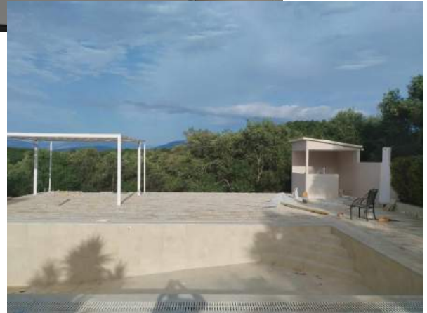
Pool area with kiosk taking shape
