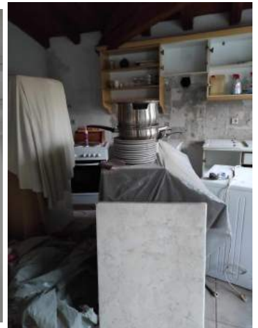
Working in kitchen area
