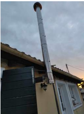
New stove pipe
