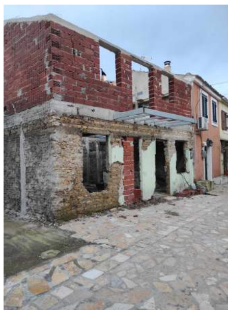
Work stopped temporarily
