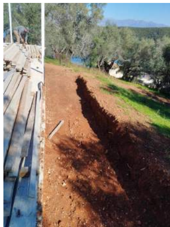
Trenchwork for patio extension
