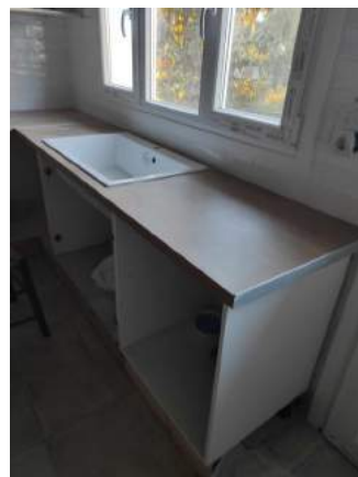
New surface and windows
