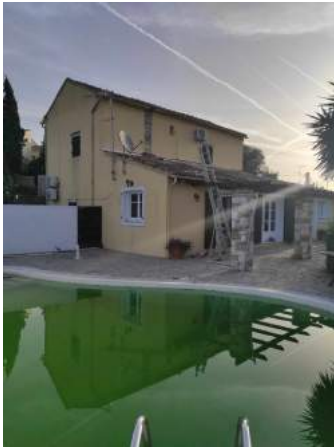
Up for roof repairs
