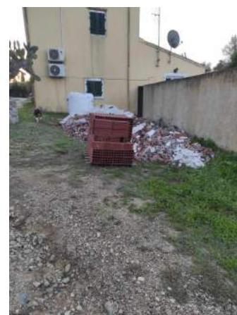
Debris out from interior
