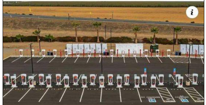
cowboystatedaily.com Largest EV Charging Station In World Powered By Diesel-Powered Generators
