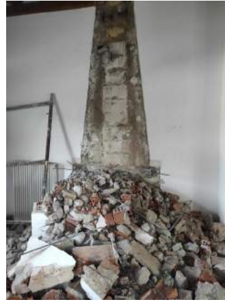
End of the fireplace
