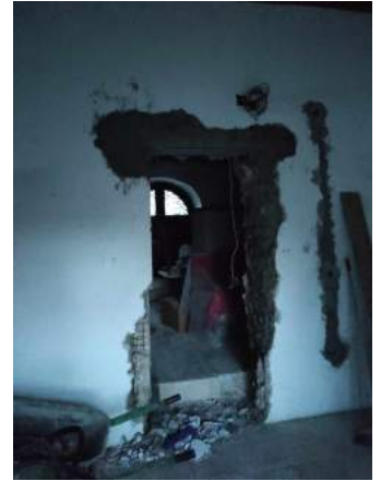
Making lounge doorway wider
