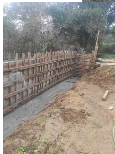
Large retaining wall
