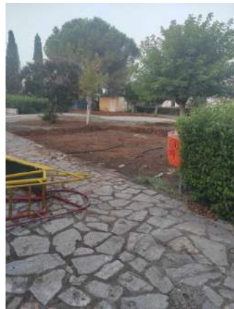
The main kids' playground being redone
