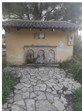
Water for the Community
