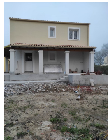
Windows rear door fitted
