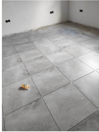
Start of floor tiling January
