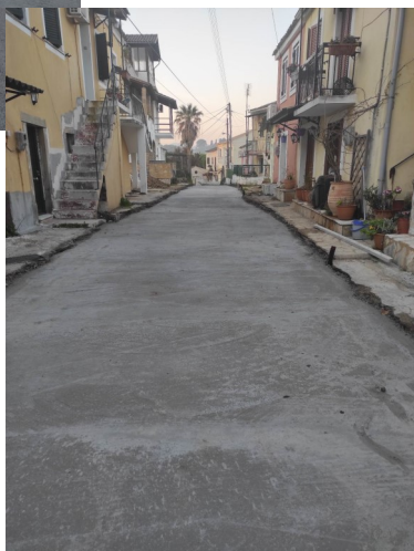
New Highway prior to flagging >
