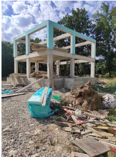
July Ring beam in place
