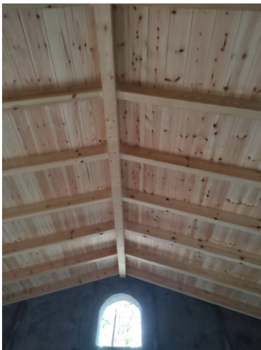
September Cathedral roof
