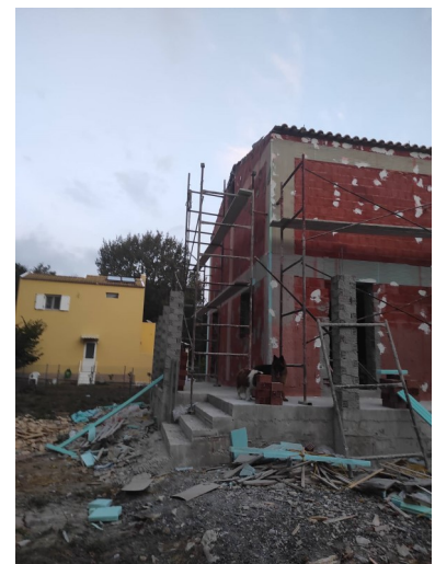
September Making good this side
