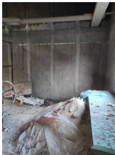
September All lines on interior done
