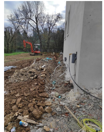
January laying to soak away
