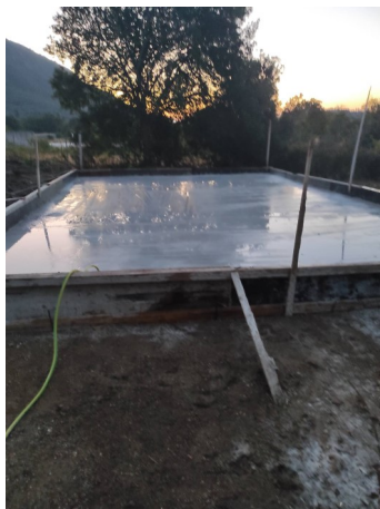
July bases finished
