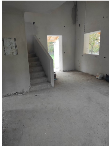
December stairs electrics plaster
