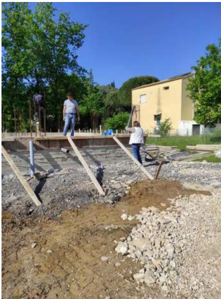
Pipes going in
