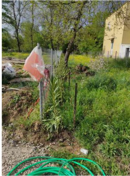
New fence line
