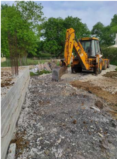
Digger is back
