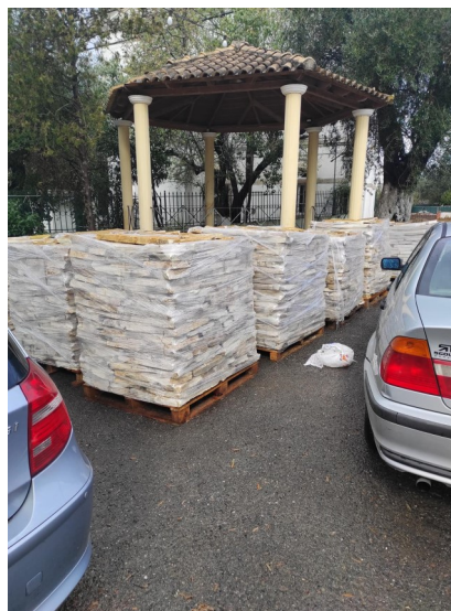
Slabs waiting to be laid
