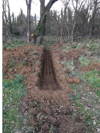
Runoff on neighbour's land
