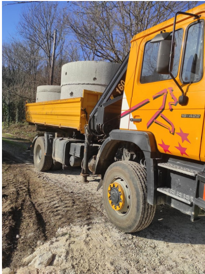
Delivery of prefabricated concrete
