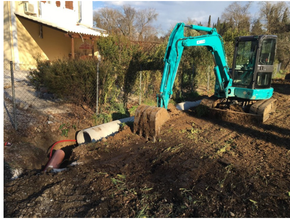
Laying of culvert
