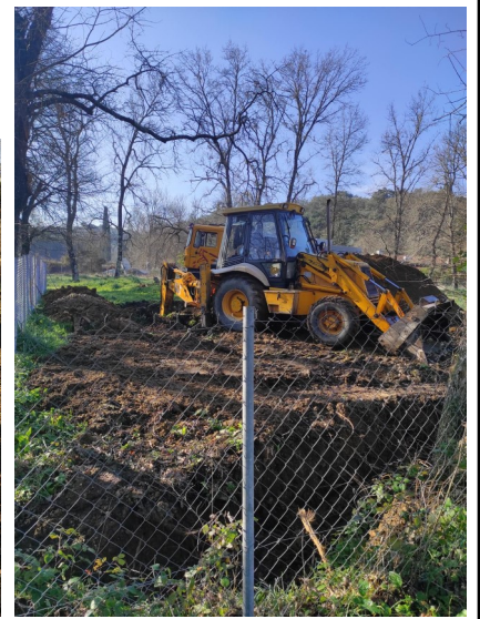
Final digging for soakaway
