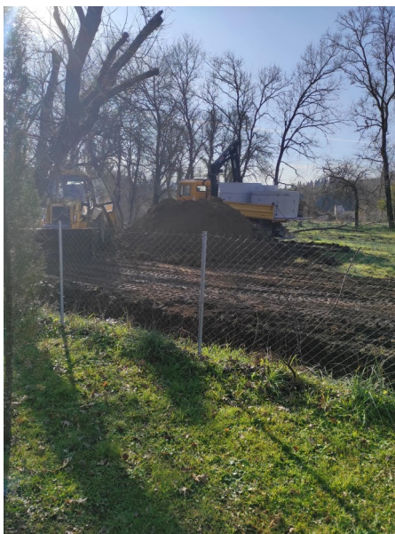
Cylinders to final location
