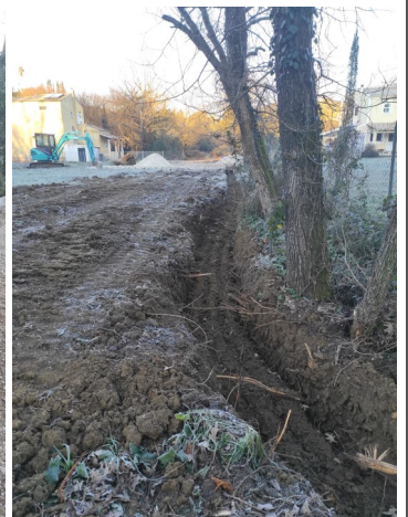
End of drainage ditch
