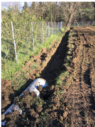
Extent of culvert in ditch towards Amazon
