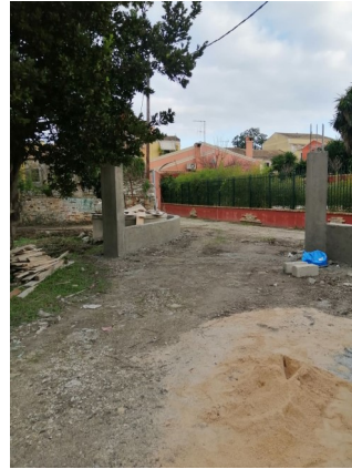
A new wall in Parados Street >>
