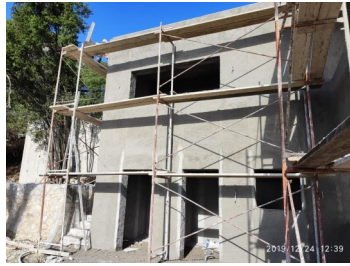
Scaffolding for plastering and painting
