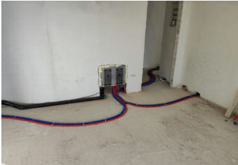
Starting to install central heating
