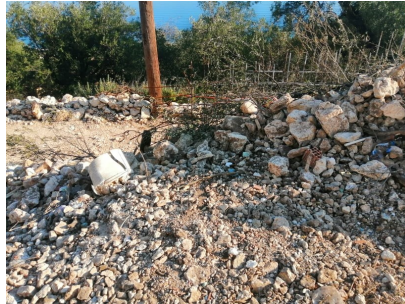
Foundation for further stonework
