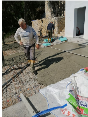
Laying screed for artificial grass
