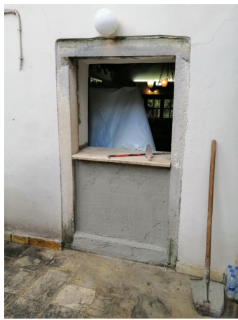
Window replacing kitchen door
