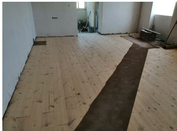
New floor main house
