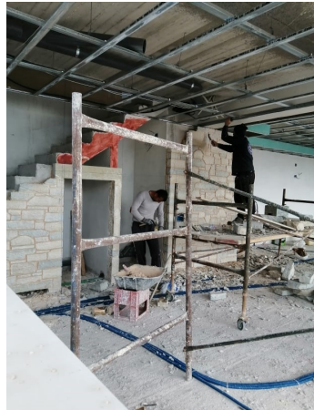
Our brilliant stonemasons
