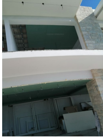
Window frames going upstairs
