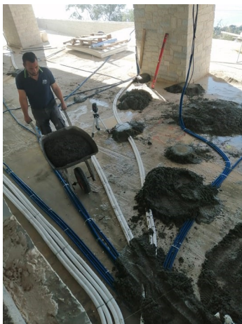
Starting the screed work
