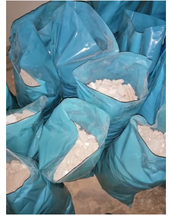
Debris from demolition
