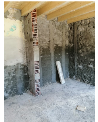
Lines for plastering
