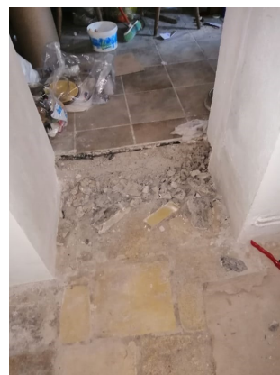
Breaking open walls
