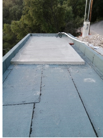
Awaiting solar panels
