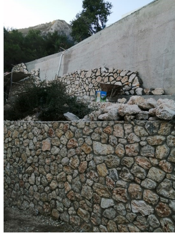
Different angle of fresh stonework
