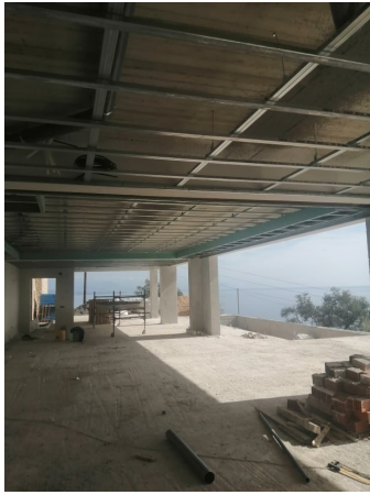
Superstructure for ceiling
