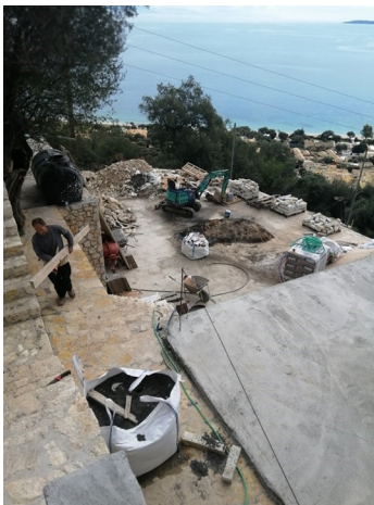
Shuttering for imminent concrete
