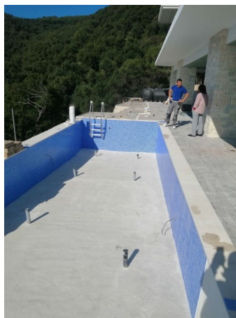
Pool sides almost tiled
