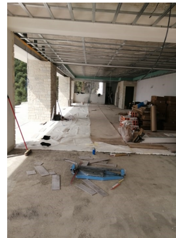
Covering the tiles for protection
