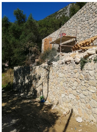
Equipment delivered up the walls
