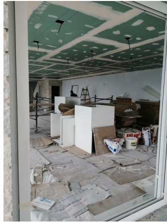
Kitchen waiting for electrician and ceiling man to depart
