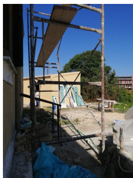
Scaffold for serious remedial
