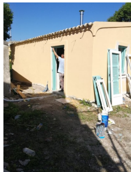
Paint job drying in fine weather
