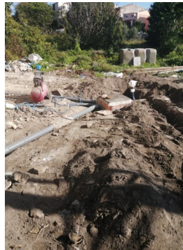
The builders have not nicked my compressor
