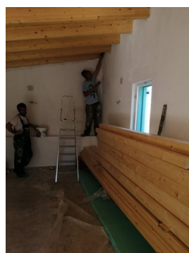
Painters applying finishing touches
