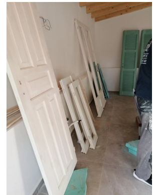
Practically finished woodwork
