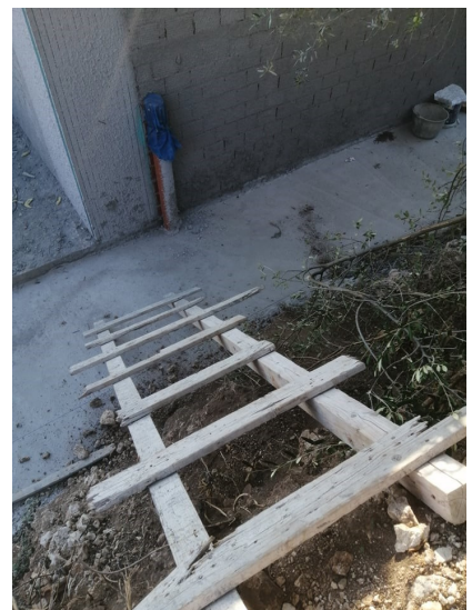
Workers' ladder to front,
