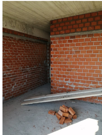
Inner walls complete upstairs
