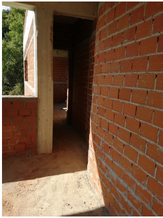
Curved wall to laundry cupboard
