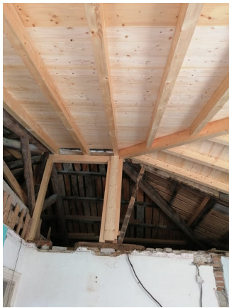
New ceiling abutting neighbour
