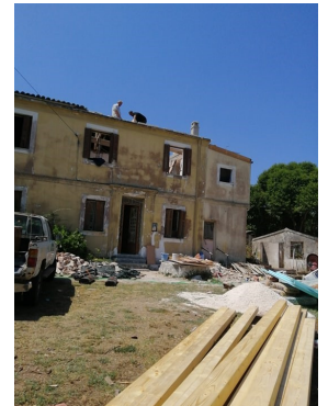
Working on roof of main house
