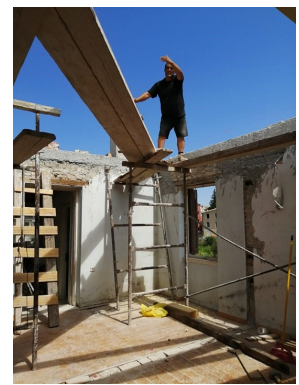
Hot work in August
