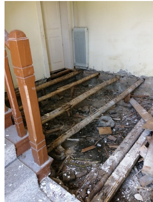
New concrete floor to go in
