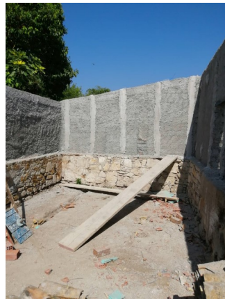
Doing the lines
