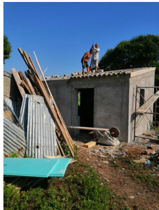
Execution on a roof
