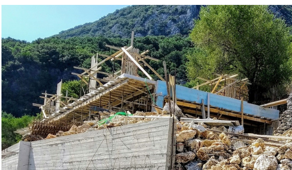
Shuttering First Floor
