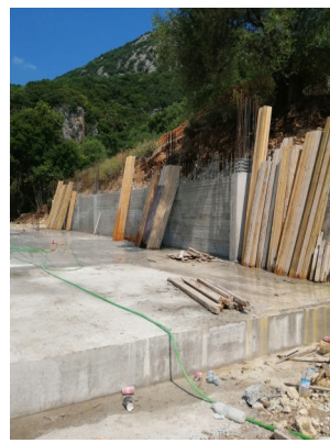
Keeping the base damp in hot conditions to stop cracking
