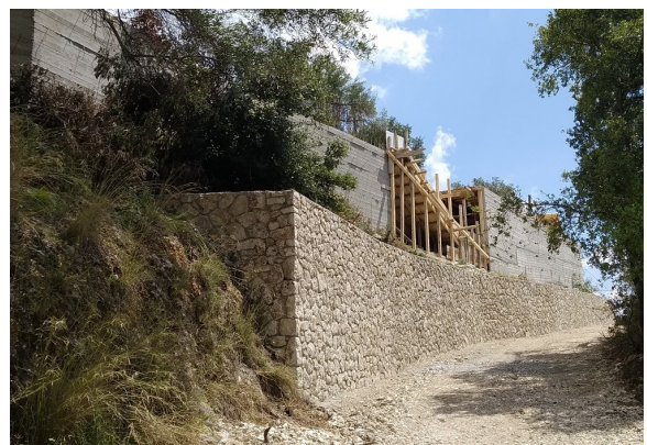
Completed stone wall aside lane
