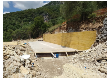
Pre-base with shuttering for Villa >
