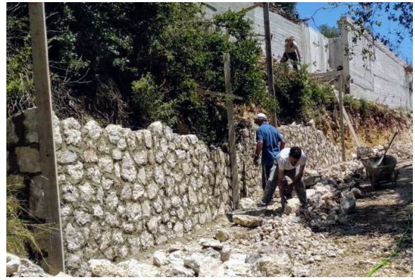
Lower stone wall construction
