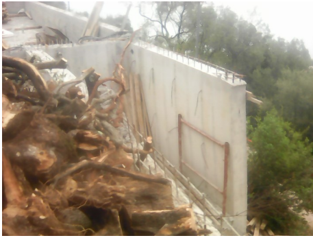
Pump room chamber
