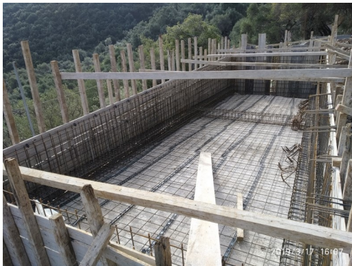
Steel in place
