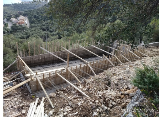
Shuttering for pool
