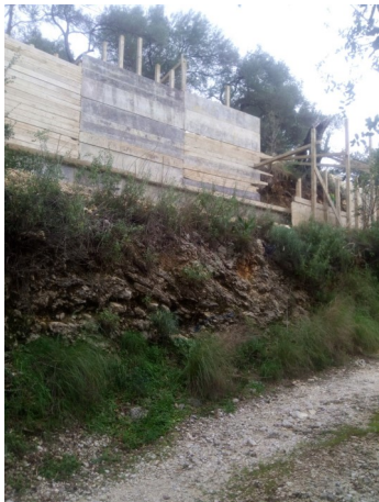
Lower wall placement
