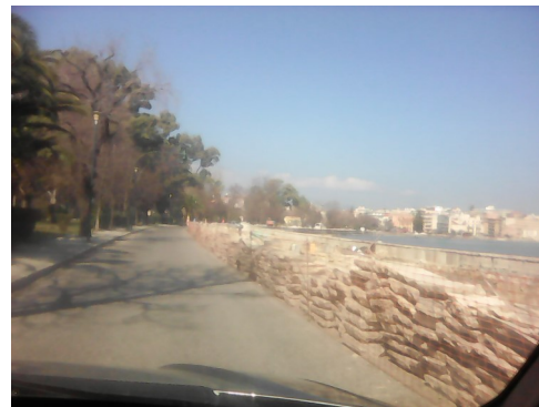
New roadworks at Garitsa <
