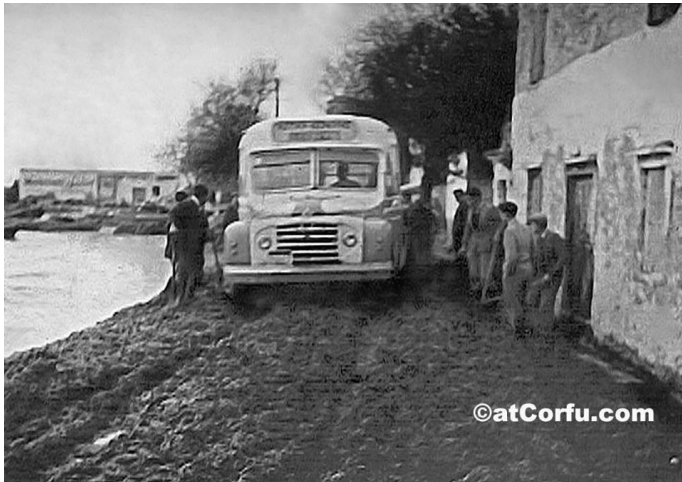
Benitses 1960 seaweed blocked the road
