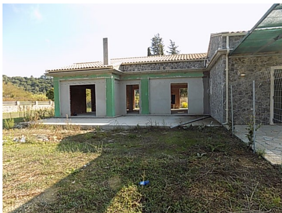
Casco Stone Villa awaiting finishing
