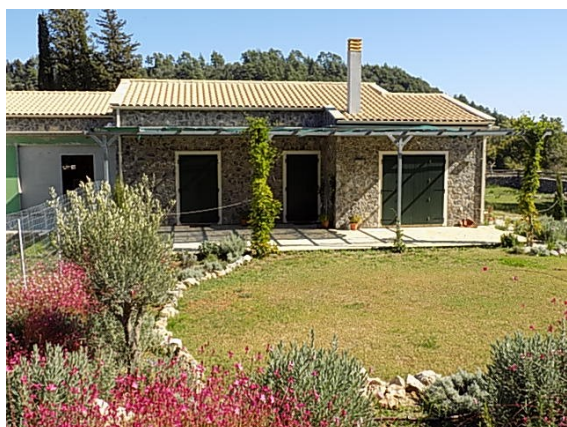
Casco Stone Villa as it could look on completion
