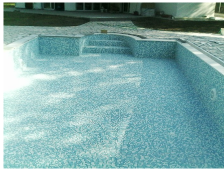
Lots and lots and lots of grouting
