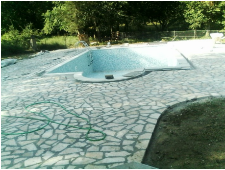
Careful attention to tiling
