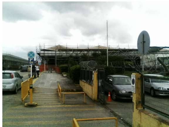
New works at the airport <
