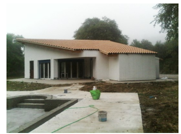
8 Pool screed with insulation
