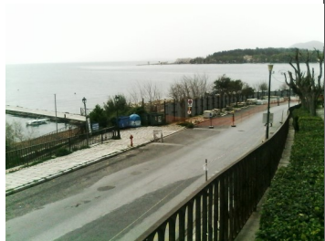
Works at Garitsa bay
