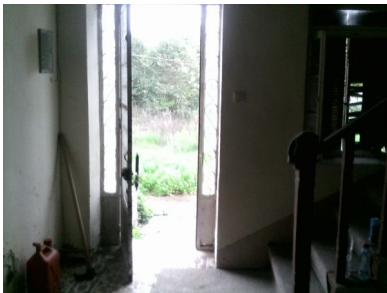
Attention to doors
