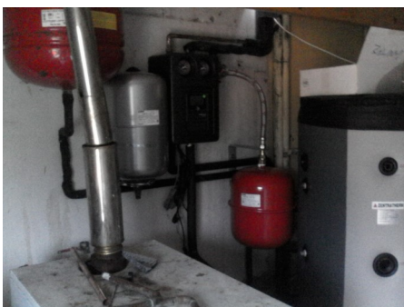
Replacing poor heating systems
