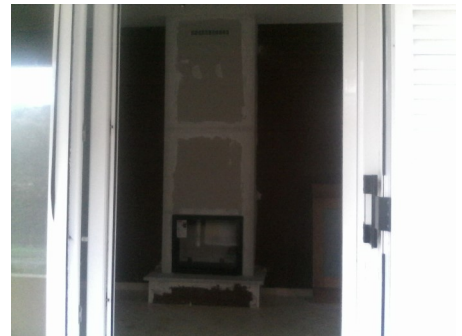
Incorporating new fireplace in existing home
