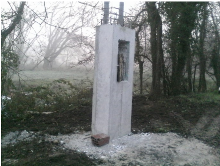
Awaiting the poles
