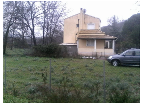
New shed from further off
