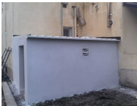
Shed extended to enclose exposed piping
