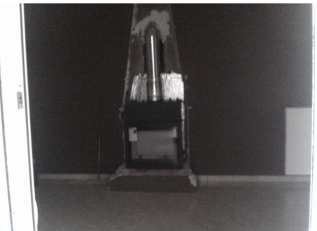
New Woodstove to chimney installation
