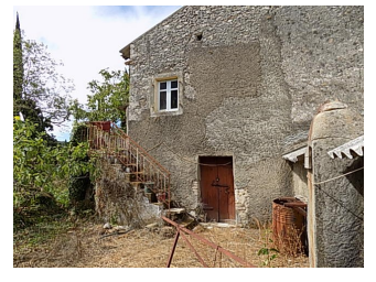
Kamara Corner House side
