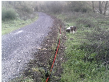
Foreman inspecting new water pipe
