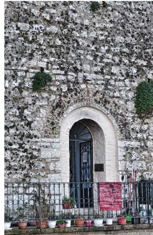
Set in the seawall
