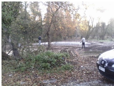
Steelwork for pool environs
