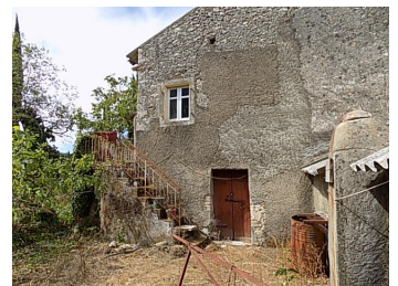
Kamara Corner House Side
