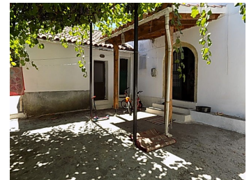
Pergola House Front 2
